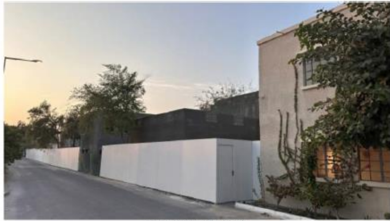
Ongoing renovation work at the village
